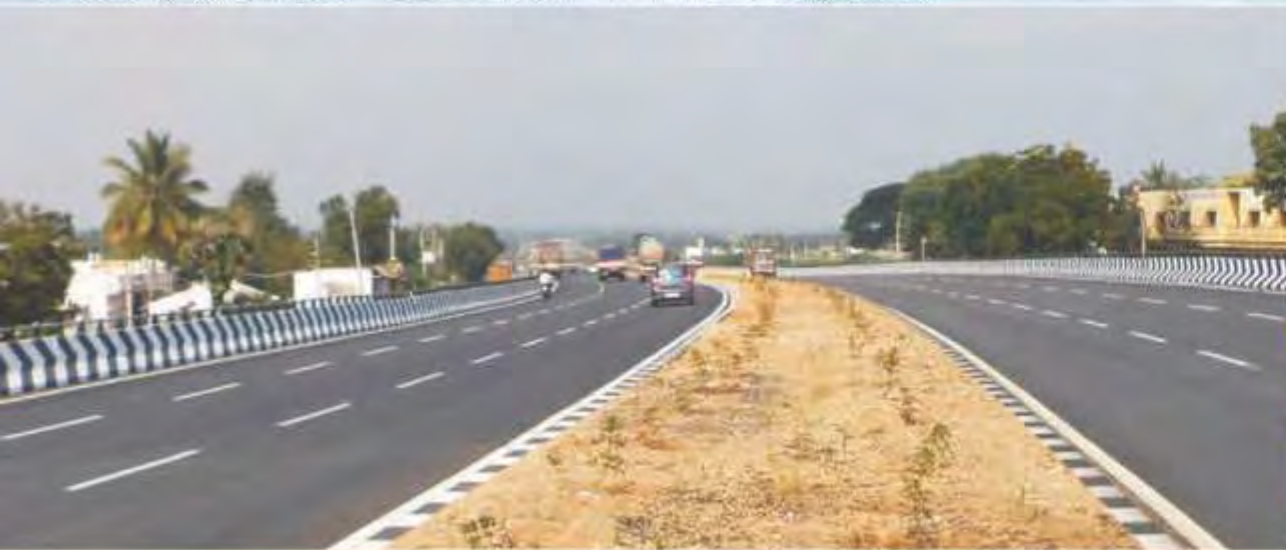
Widening of Mumbai - Goa Road & Vadkhal - Alibag Road.
